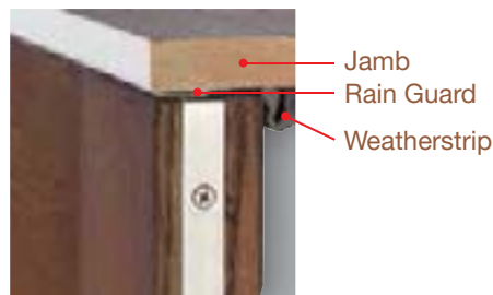
Top of door; exterior view.
